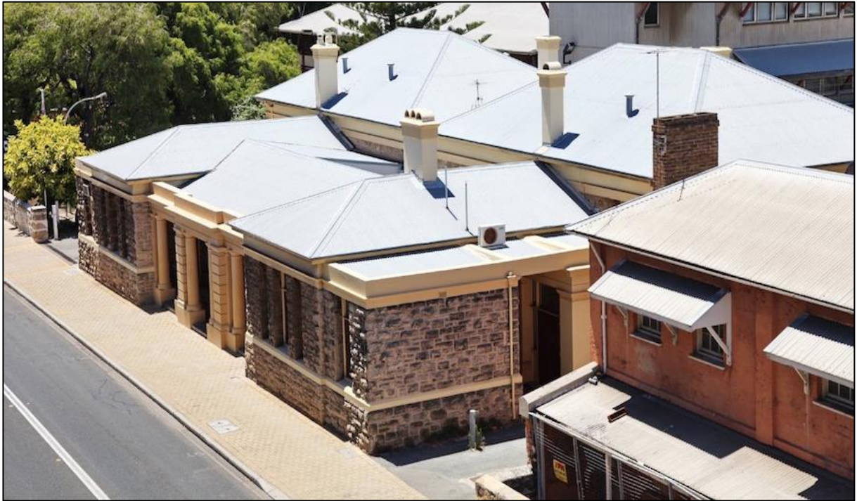
Figure 17: Fremantle Police Station Complex
